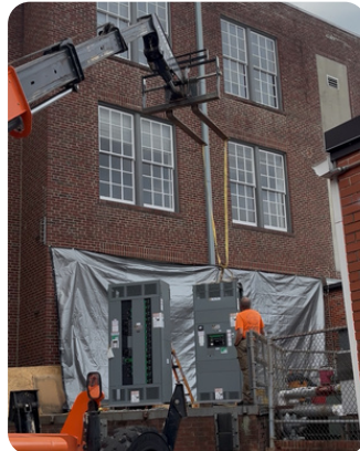
Photos from replacement of the switch gear (2025).
